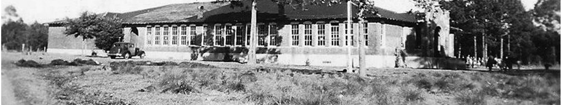
The old Holley Elementary School was once the hub of the community. The building was demolished years ago, and the only remaining images are in memories and old photographs such as this one.
